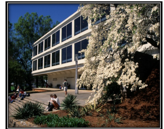
R.C. Wilson Pharmacy Building
